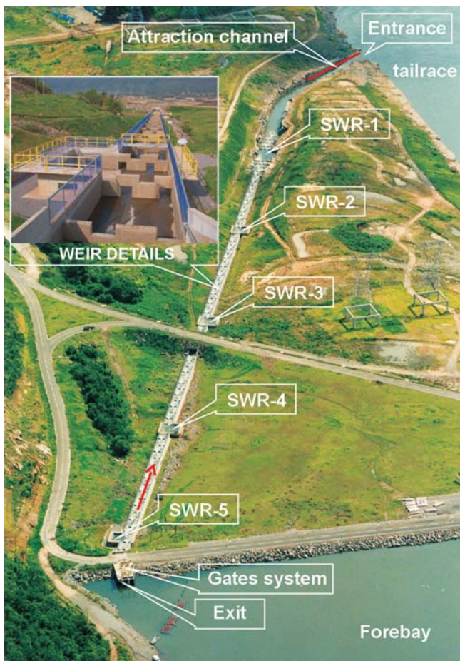
Fig. 1. Overview of the fish ladder and details of the weirs. SWR = Still Water Rest.
